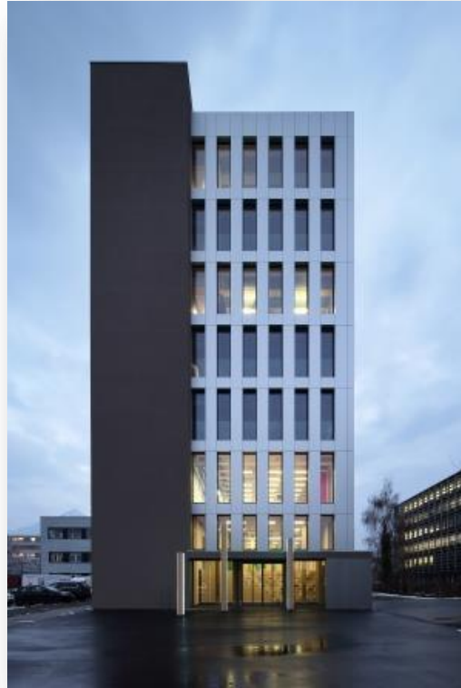
17,222 sq.ft. (1,600 m 2 ) pilot building for CREE's Life Cycle Tower building method. 8 th. Storey building with construction one floor / day
