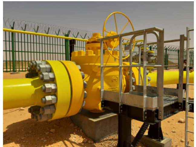
20°CL. 2500 High-Pressure Ball Valve Onshore, Algeria
